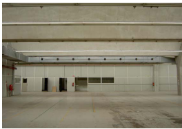
weverij \ textile mill De Ploeg in 2008 [foto MS NvV]
